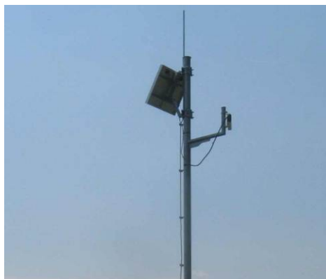
Slika 3. Fotonaponski paneli i antena WiFi AP Figure 3. Photovoltaic panel and WiFi AP
