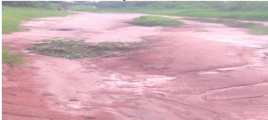
Plate 5: Erosion at site E
