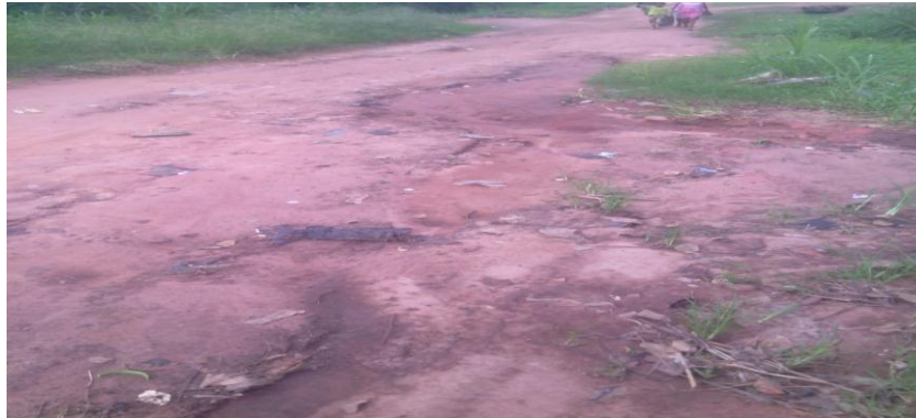
Plate 7: Erosion at site G
