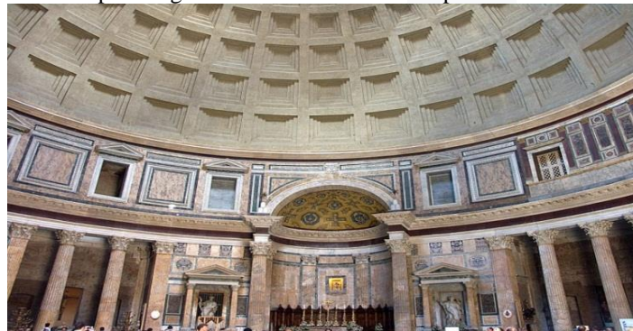
The photo 1. The Pantheon in Rome is an example of Roman Concrete Construction, [2].
